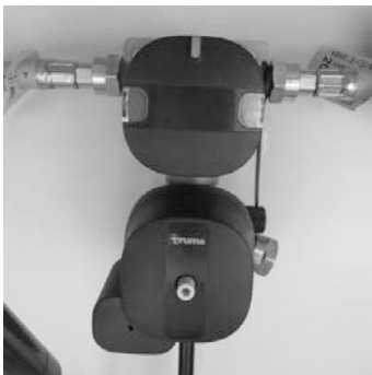
Fig. 109: DuoControl CS gas supply
