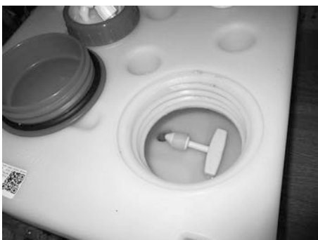
Fig. 92: Drain plug in the fresh water tank
