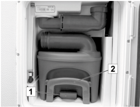
Fig. 154: Waste holding tank in the disposal shaft
