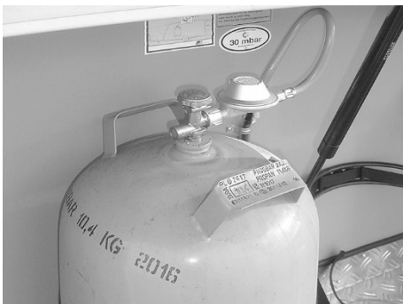
Fig. 107: Gas bottle with pressure reducing valve
